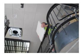
The owners found a great location, but could see noise was likely to be a problem. The construction materials were predominantly glass and concrete; materials that cause sound to bounce around and make a space 'noisy'. This venue was a typical example of where sound absorption needed to be introduced, whilst keeping the raw rustic look that the owners wanted.
