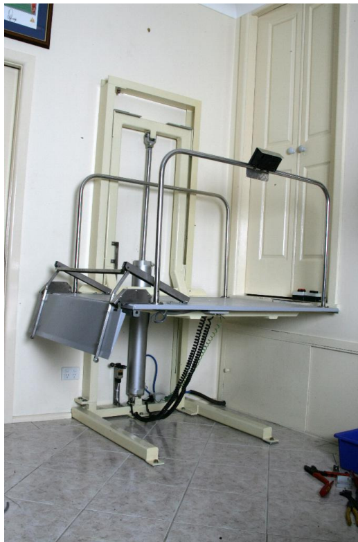
Fig 3- The new lift with out the covers showing the SMC CG1 pneumatic cylinder
