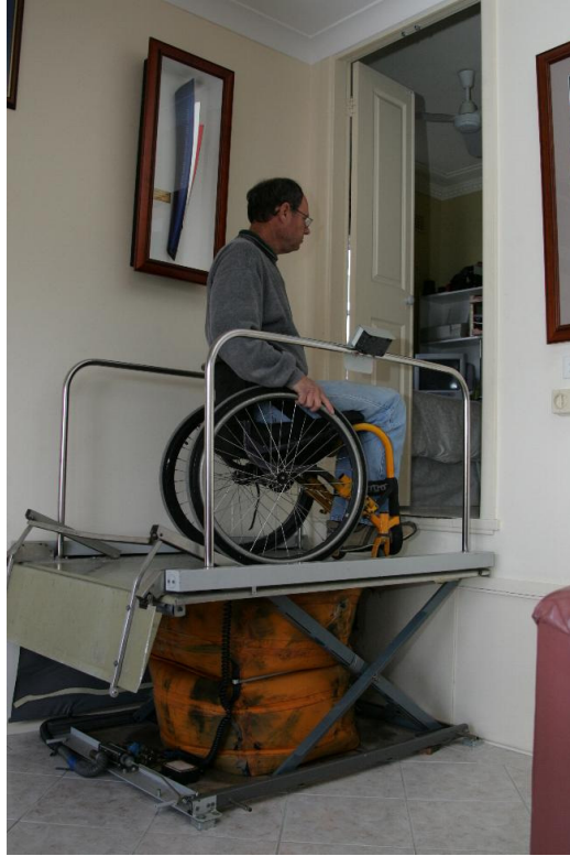
Fig 1- The old lift with an air bag could not longer reach the top level
