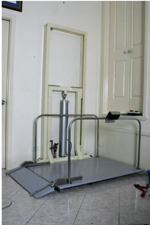
Fig 2- The new lift during construction showing the SMC CG1 cylinder
